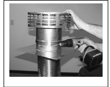
Flex Termination Cap Installation
