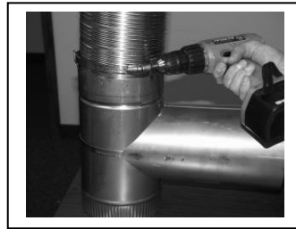
Flex Tee Installation
