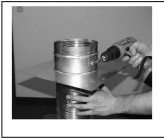
Flex Support Plate Installation
